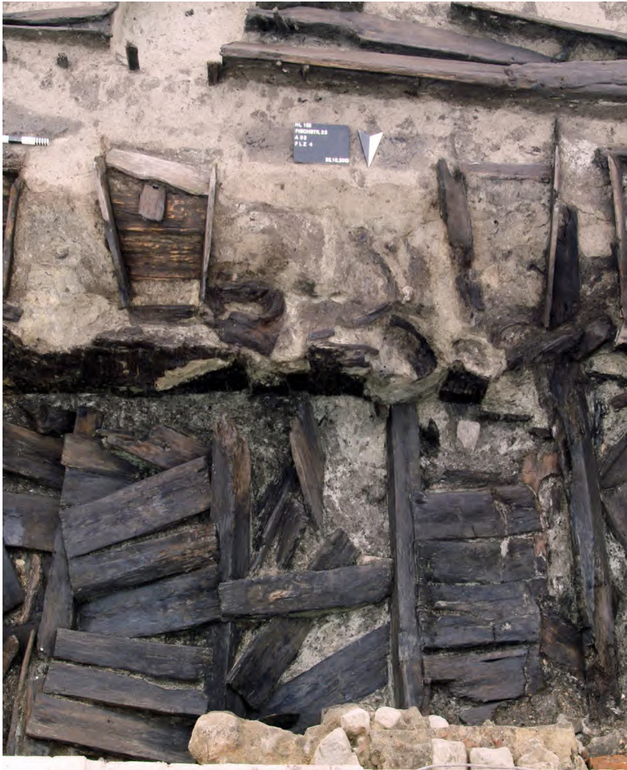
Fig. 10 Clearly visible are the trapezoidal air vents / light shafts of this cellar excavated at Alfstraße 23, Lübeck, and built in 1166 AD (photo: Rieger 2019, Abb. 88).
